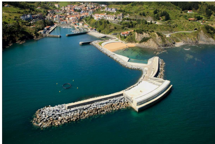
Illustration 2 Aerial view of the Mutriku Wave Plant
